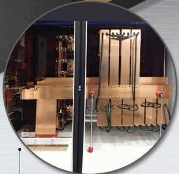
Picture showing the Inverter & Capacitor arrangement of AMELT Induction Power Supply .
